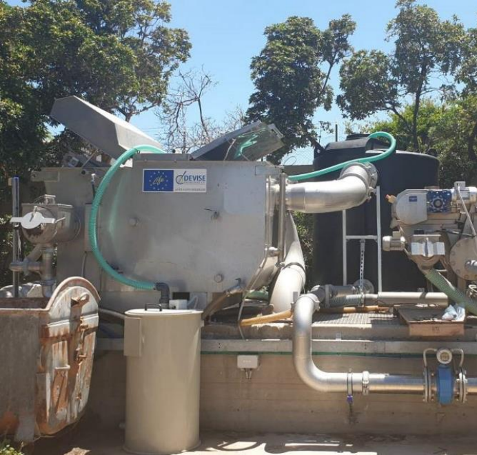
Microscreen with feeding line and dosing system
